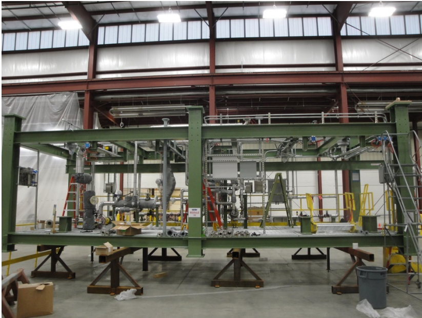
A single completed module
