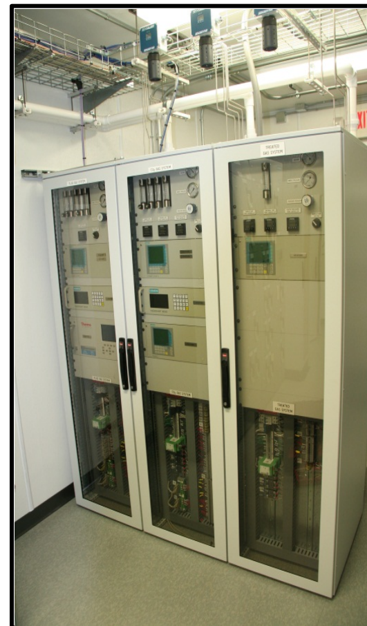
Analyzer and sampling panels
